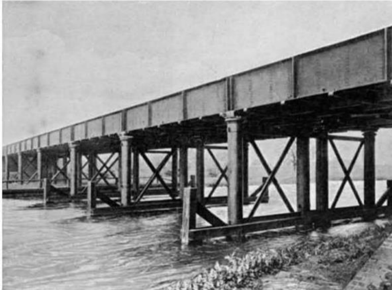
Figure 1: Photograph showing 1856 bridge
