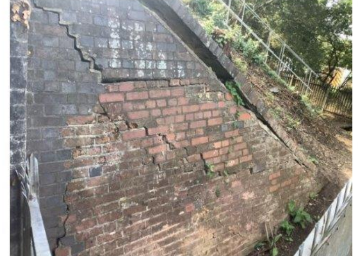
Photo No 8 - Low Mileage Downside Wingwall - 22/09/2022
