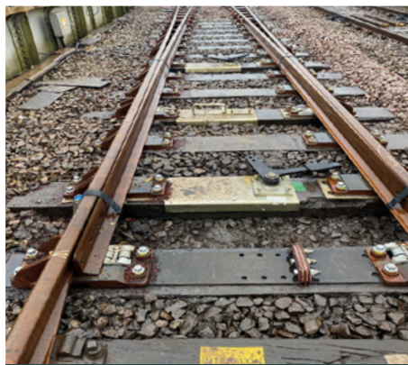
Figure 8: Carmarthen installation with Excalibur Screwbolts.
