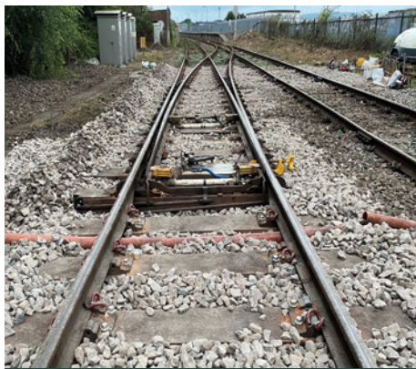
Figure 7: Ninian Park installation with Excalibur Screwbolts.
