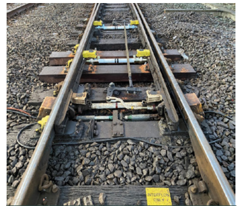
Figure 9: Carmarthen installation with Excalibur Screwbolts.
