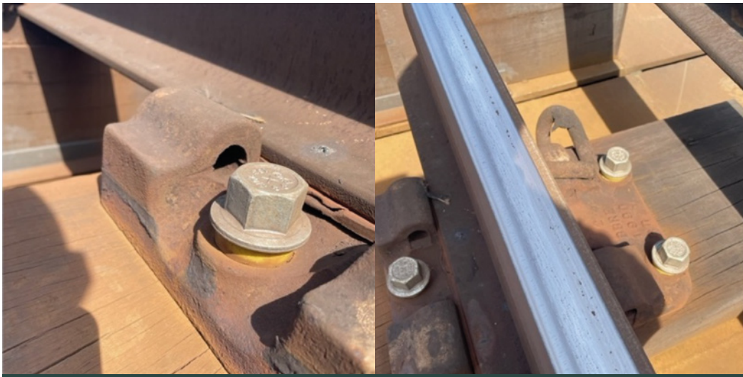
Figure 13: Excalibur Screwbolts firmly seated.
