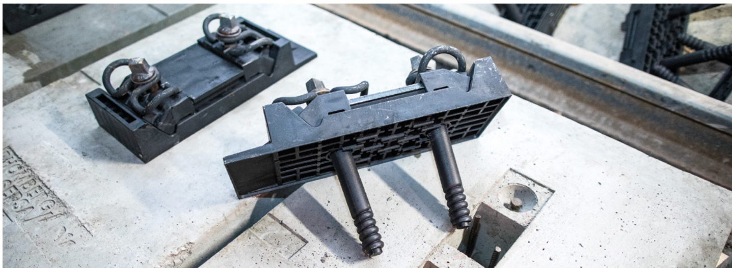
Figure 2: Vossloh DFF 300 RS before assembly of track panel; also visible are the grouting pockets on top of the IVES blocks.
