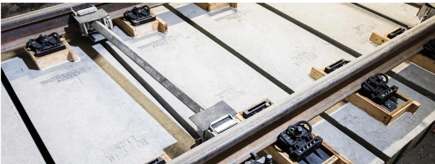
Figure 3: Track adjustment system RhoFAS supporting the track panel, placed on IVES blocks. Formwork installed around the fastening system. (Copyright RSRG).
