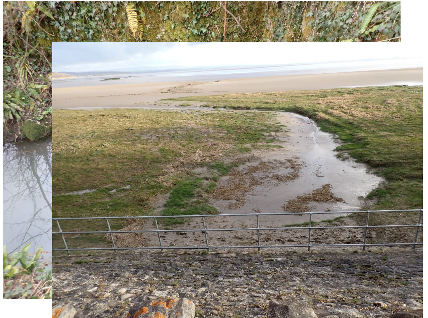
Seldom Seen Culvert (Images: RAIB)
