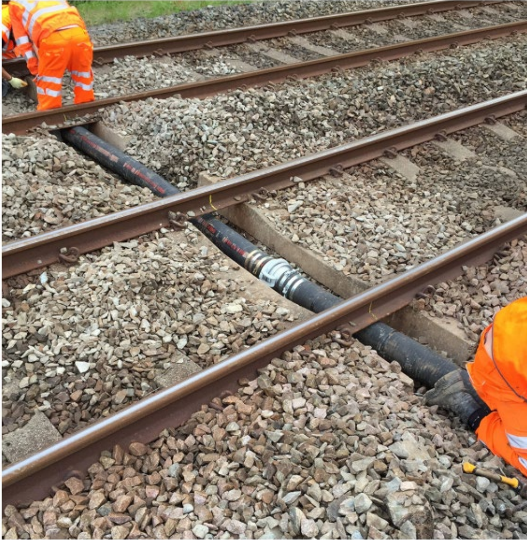
Installation of Tempory Pipe (Image: Network Rail)
