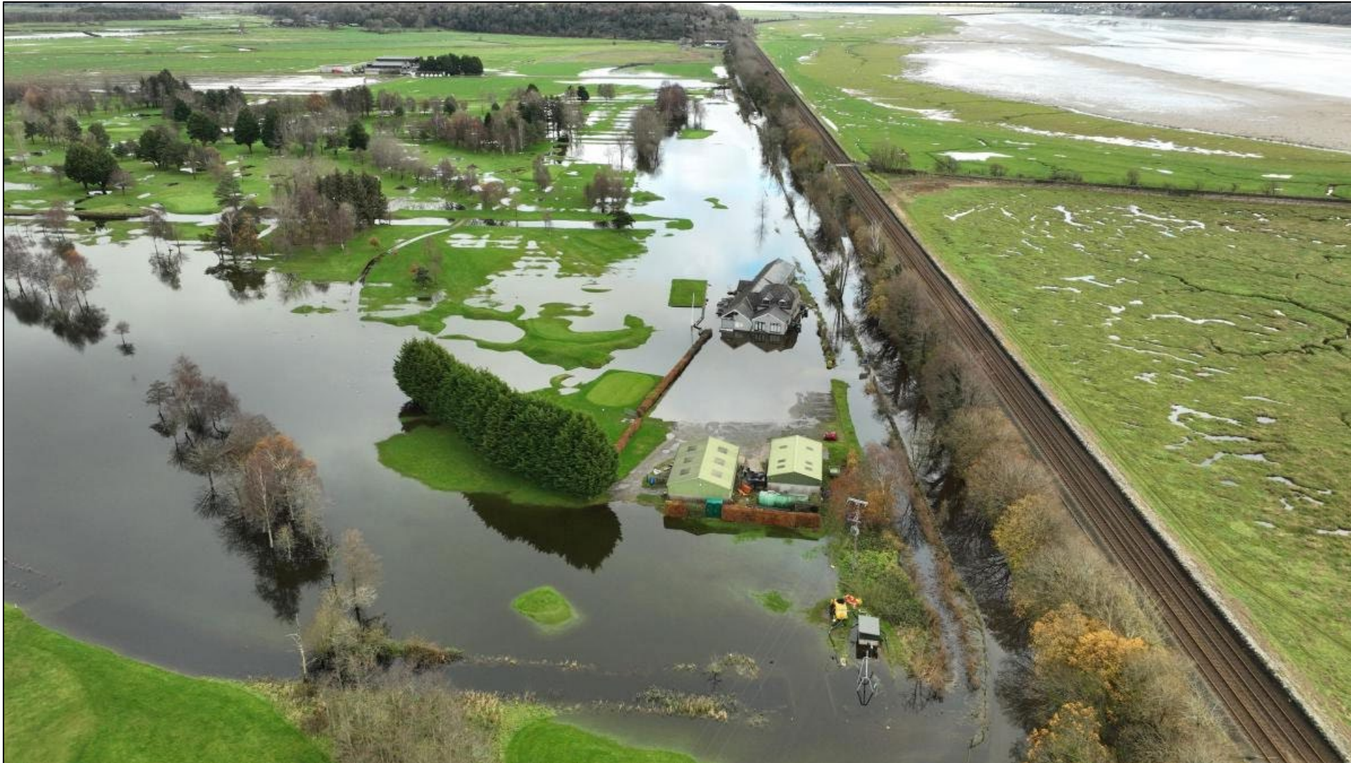
Flooding at Grange-over-Sands Golf Club (Image: Leslie Micklethwaite)
