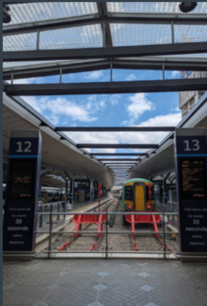
2 completed platform installations at London Bridge (Photo courtesy of Molly Dalton).
