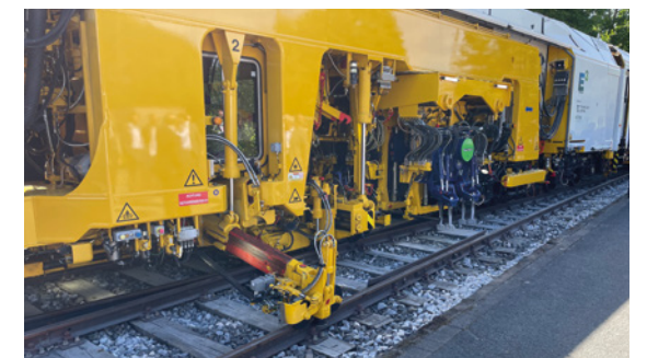
Plasser and Eiffage demonstrate fully automatic (no operator) switch and crossing tamping.
