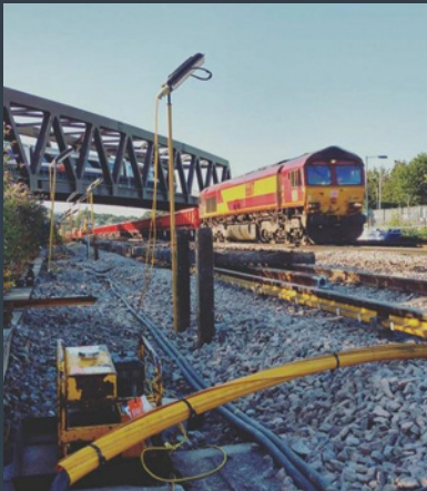
My first S&C installation waiting to kick off at New Cross Gate (Photo courtesy of Molly Dalton).
