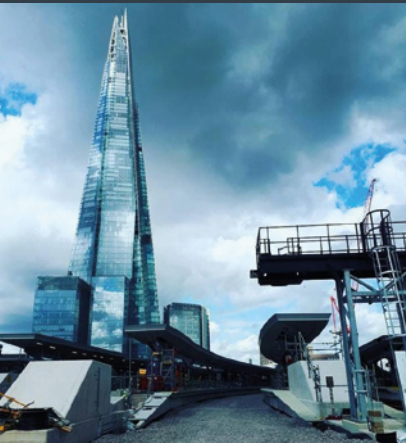
Lovely basestone installation at London Bridge Thameslink project awaiting track installation, a rare sight to see a platform without any track (Photo courtesy of Molly Dalton).
