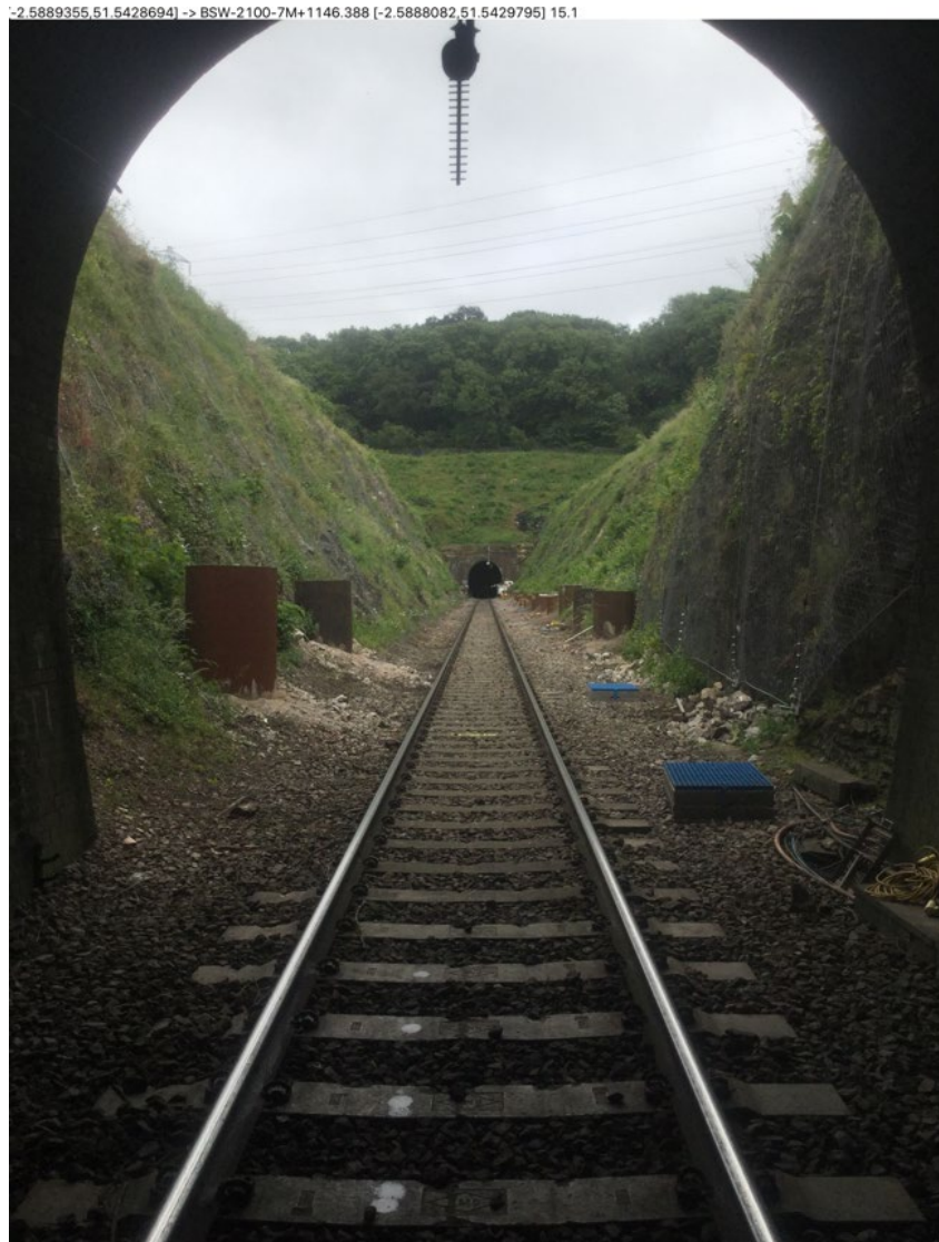
Mid Construction Visit looking to short tunnel
