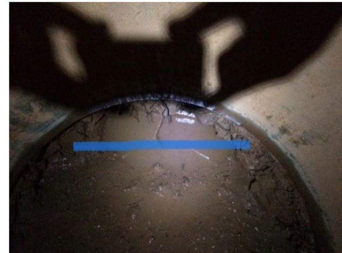
Silt removal to permit CCTV surveys – note crown indicated in blue
