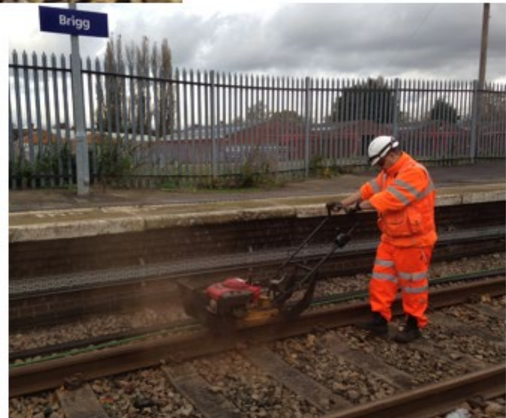
Photos: Network Rail
