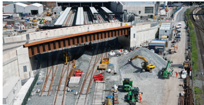
Figure 5: Permanent Way Construction Station Area and East Ramp (Photo courtesy of Babcock).
