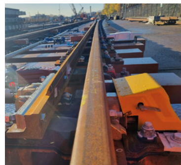
View from toes of Woodwalton 1158 points, a trial site for composite bearers on NR60 Mk2 S&C. (Photo courtesy of Dominic Meakin).
