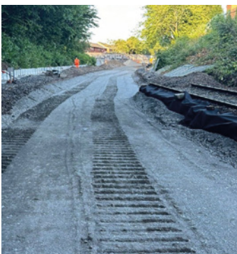
Figure 20: Formation works on the Central Curve (Photo courtesy of Babcock).
