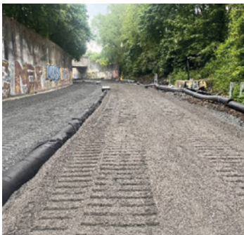
Figure 17: Summer Blockade Part 1 – prepared formation and new drainage on the Blythefield curve (Photo courtesy of Babcock).
