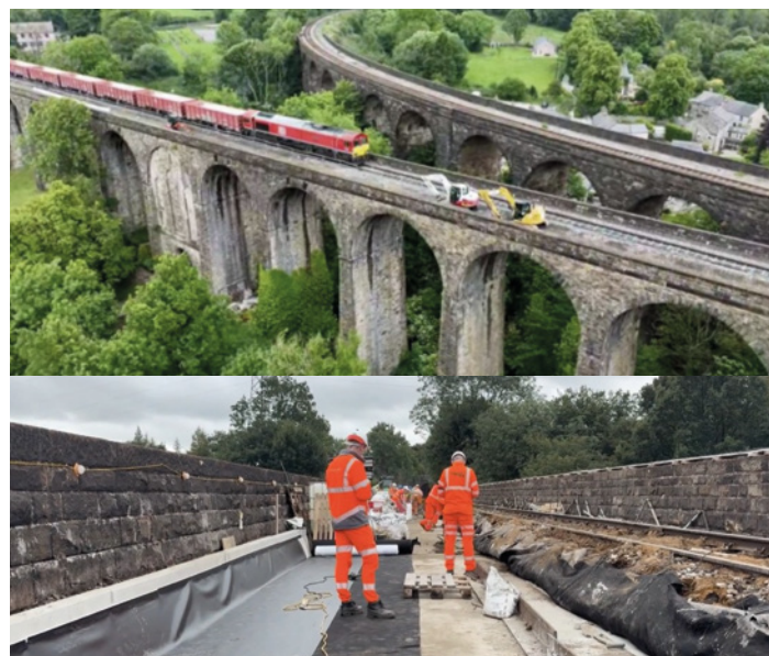
Figure 1: Chapel Milton Viaduct Derbyshire (Photos courtesy of Network Rail).
