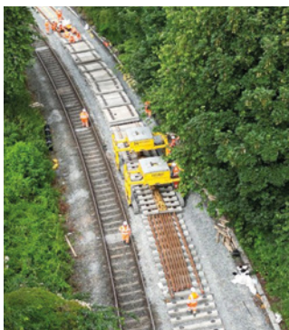
Figure 21: Track construction for the Central Reversible (Photo courtesy of Babcock).
