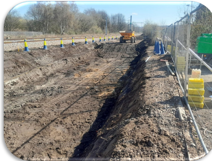
Vacuum excavation used around S&T cables and services
