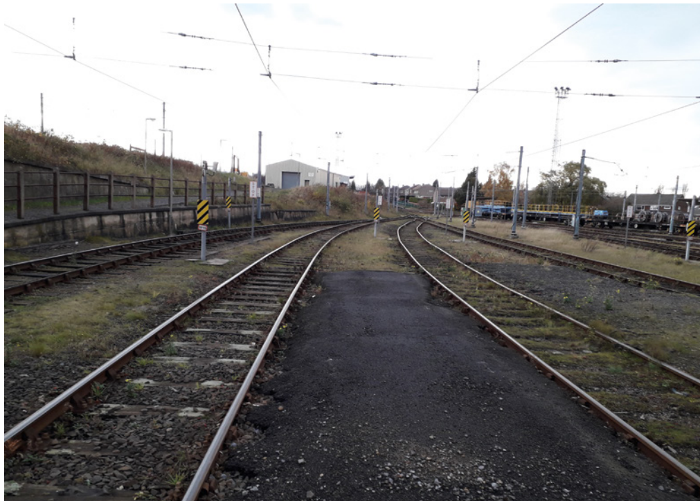
Figure 4: View facing west between existing depot road 18 and 19 highlighting the southern embankment.
