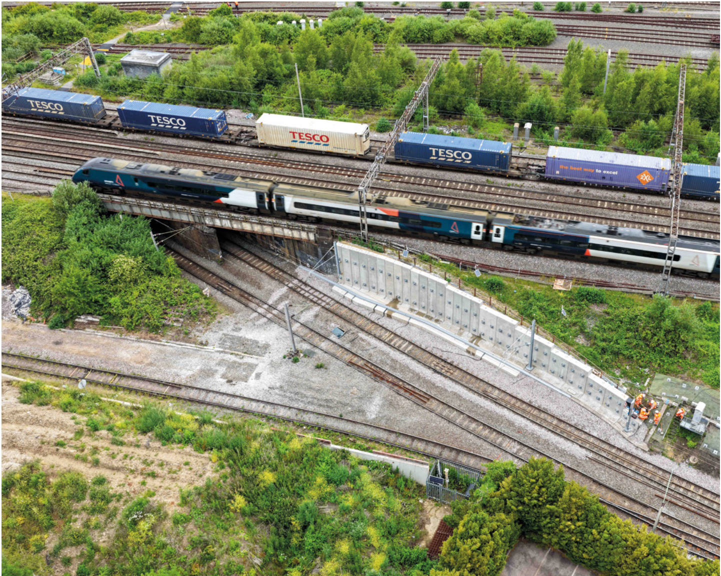
Figure 7: The completed solution.
