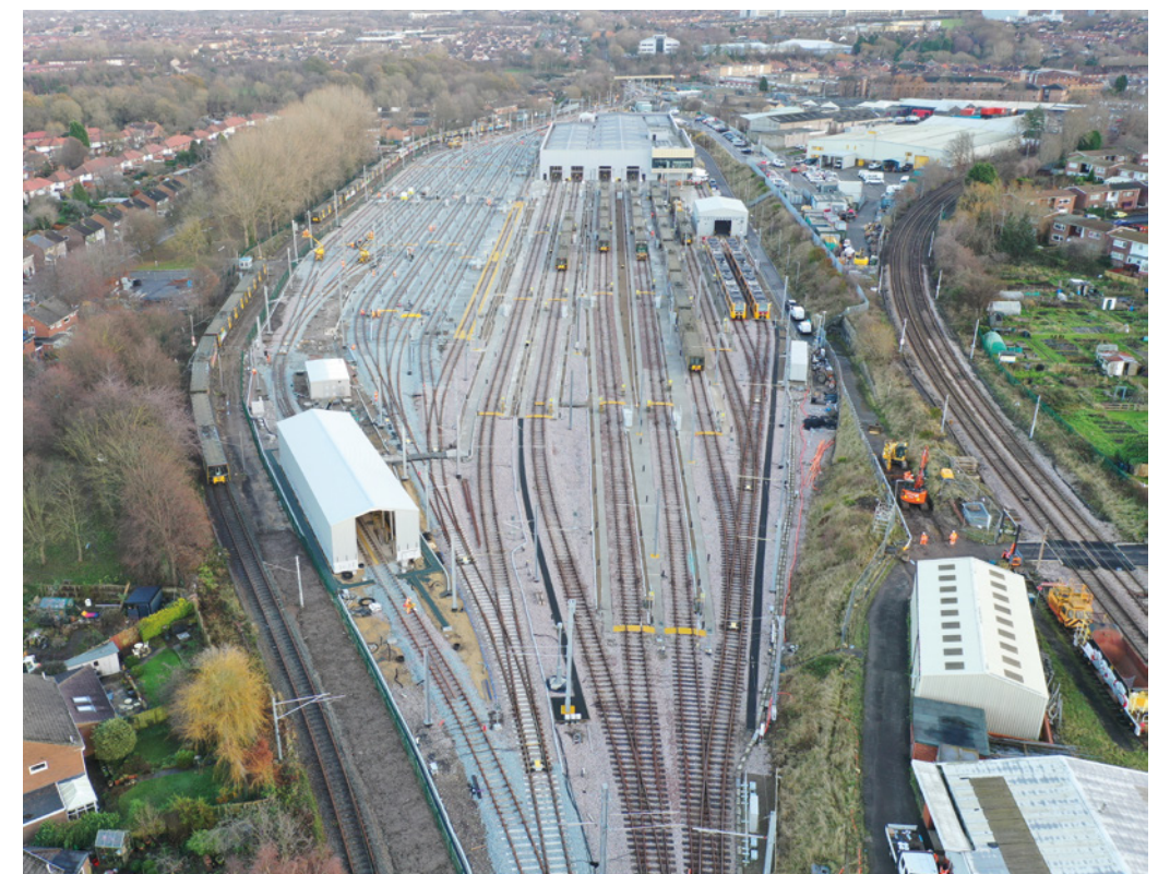
Figure 5: Eastern approach showing, from right to left, Sidings 1 to 17 (Image courtesy of Stadler Rail).
