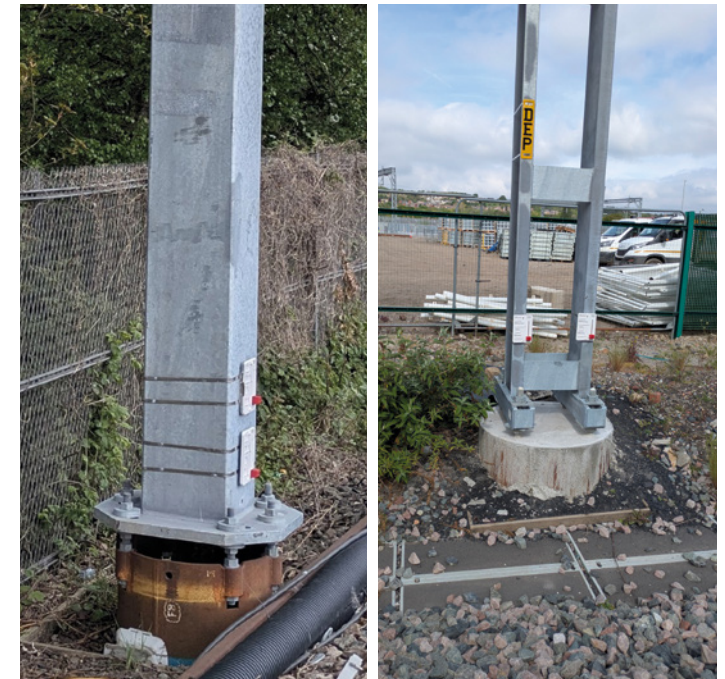
Photograph 5: 610mm CHS piled foundation (left) and Photograph 6: 1000mm diameter concrete auger foundation (right).
