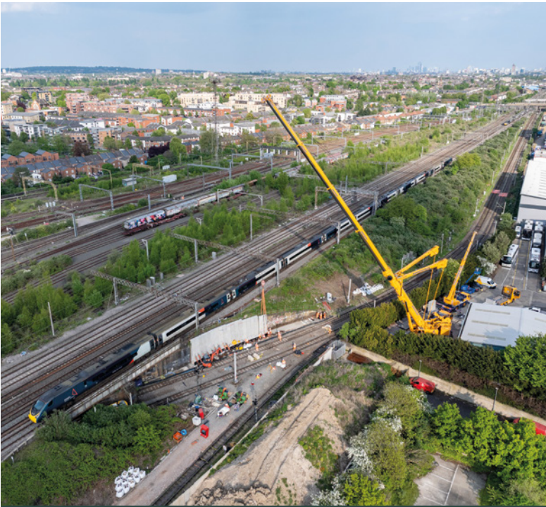
Figure 6: Construction of the toe retaining wall under live railway conditions, illustrating spatial and operational constraints.
