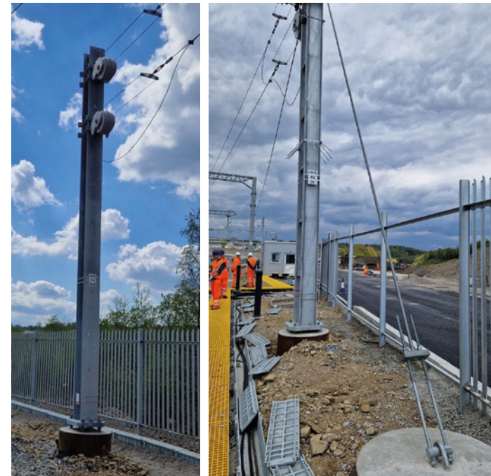
Photograph 3: SSA mast (left) and Photograph 4: Mast with back tie (right).
