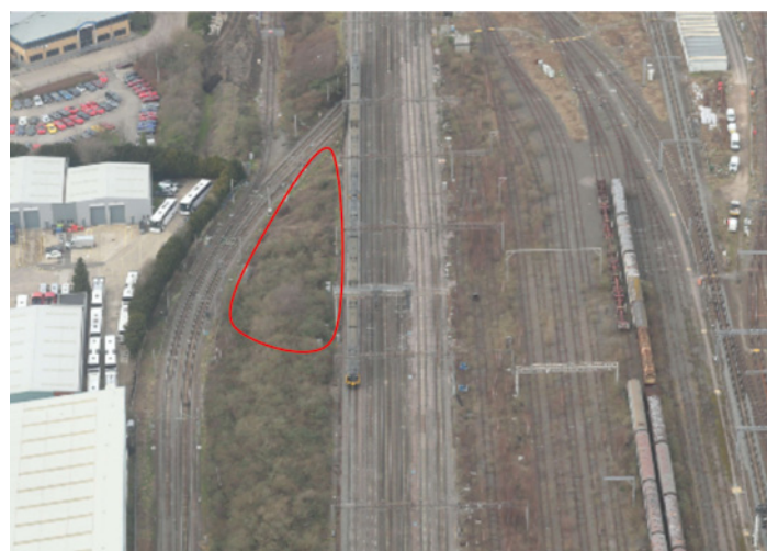
Figure 1: Location plan showing Harlesden Embankment on the West Coast Main Line, including proximity to the adjacent freight route and intersection bridge.
