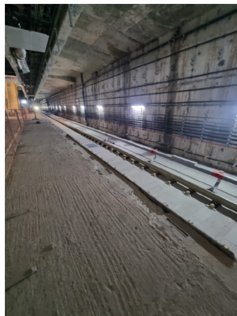
Figure 1: Platform interface works on a new station within a Mass Rapid Transit (MRT) extension. Description: Platform interface works associated with the installation of Platform Screen Doors at a new station constructed as part of an extension to an existing MRT network. While the station itself is not yet operational, the works illustrate system interfaces between track, civil structures and station systems prior to handover.
