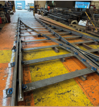
Figure 2: Assembled S&C layout under construction at KGJ Price for an oil platform project in Brunei.
