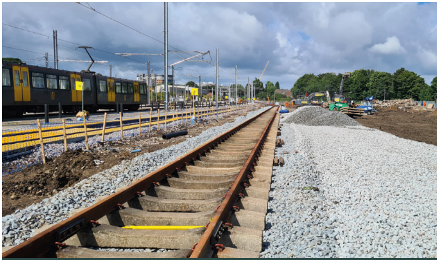
Figure 9: View facing west on Road 8 during early Stage 5 of construction.
