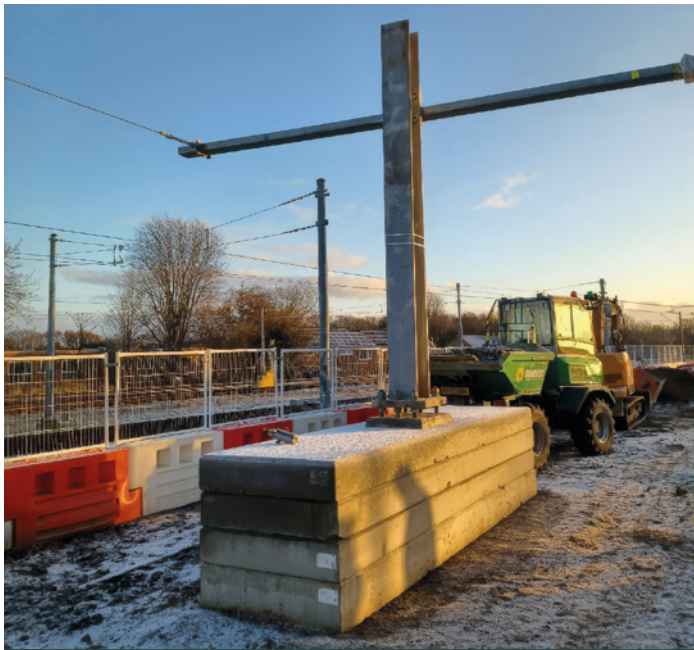
Figure 7: Bespoke temporary “biscuit” foundation used during staged construction.
