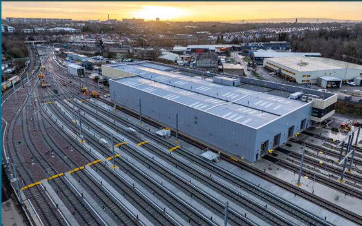
Figure 1: Modernised Gosforth Depot (Image courtesy of Stadler Rail).
