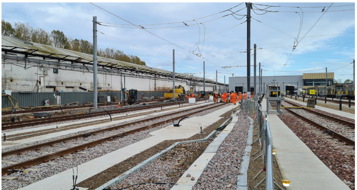
Figure 8: Proximity of retained depot infrastructure during Stage 3 of construction.
