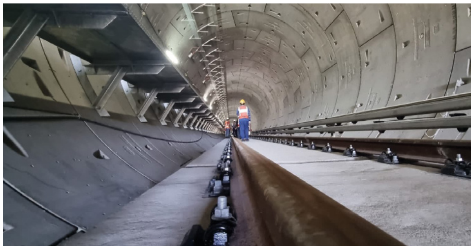
Figure 2: Tunnel inspection under constrained access conditions. Description: Track inspection and verification activities within a tunnel environment, illustrating constrained access, limited visibility and the reliance on professional judgement during rail engineering inspections conducted under restricted working conditions.
